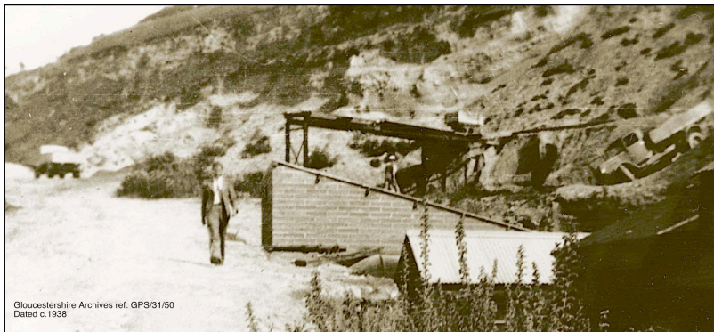
The kilns area under construction c. 1938
