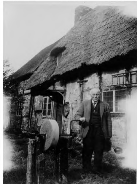
Mr Humphries at Uckington Gardens. The older market gardening houses were timber framed, with daub and wattle infill
