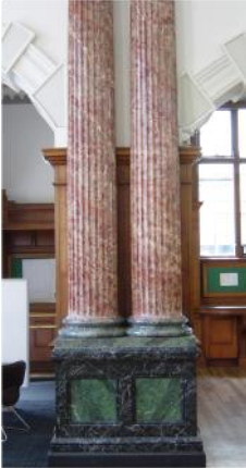
Fig.1 Pilaster in Lloyds Bank, High Street composed of scagliola .
