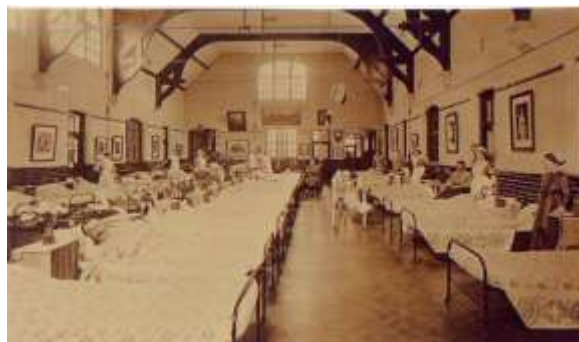
Gloucester Road VAD Hospital
