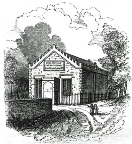
Built in 1830, the Infant School building, St. James' Square, is the oldest surviving such building in the country.
