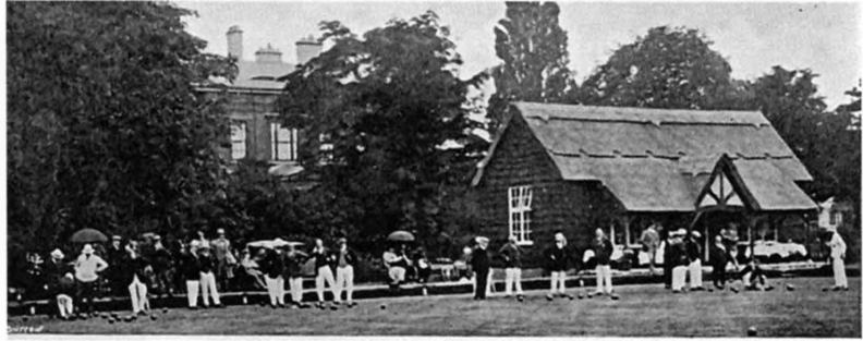
Cheltenham Bowling Club, Suffolk Square - The 'Unwin' Pavilion, destroyed by fire in 1955.
