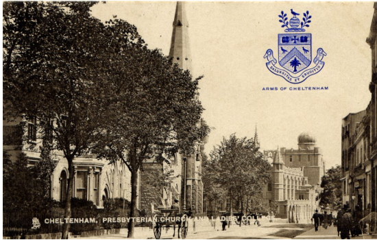
St. Andrew's Presbyterian [now United Reformed] Church, designed in Gothic style by Thomas Arnold, opened in 1885. This postcard view c1900 shows the church very much as it is today, at the heart of a thriving community close to the Ladies College and the shopping area of Montpellier.
