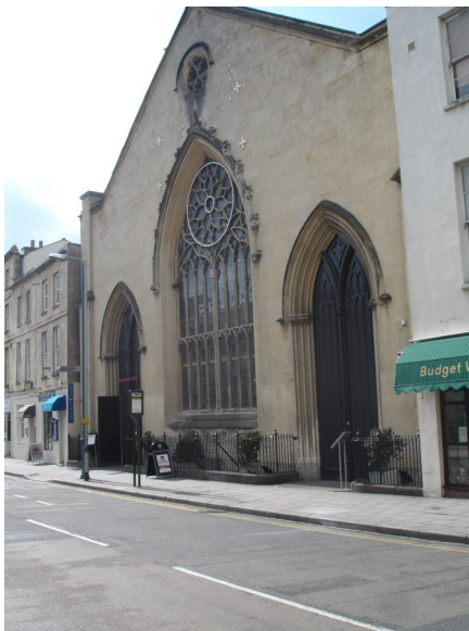
Photographed 8th September 2007, Salem Chapel now houses a bar and restaurant.
