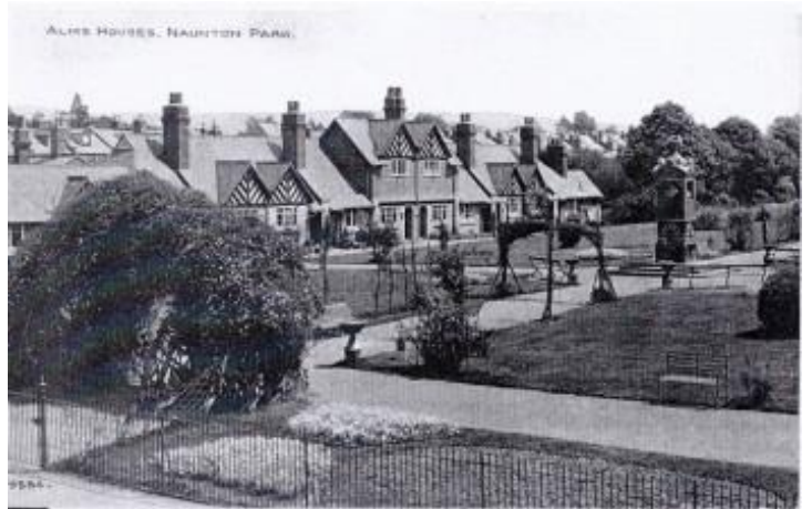
26. Hay Memorial Cottage Homes, Naunton Park. These almshouses were built in 1899, and are still in use in 2009.
