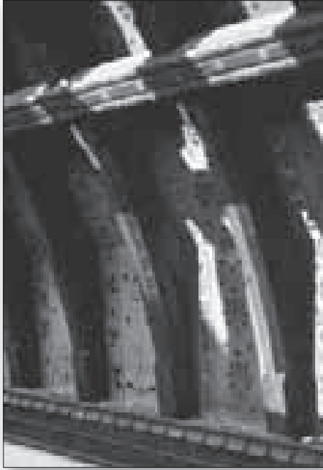
Fig. 40 Cheltenham, Westholme, the stairway ceiling
