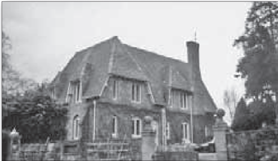
Fig. 55 Clearwell, the Hospital
