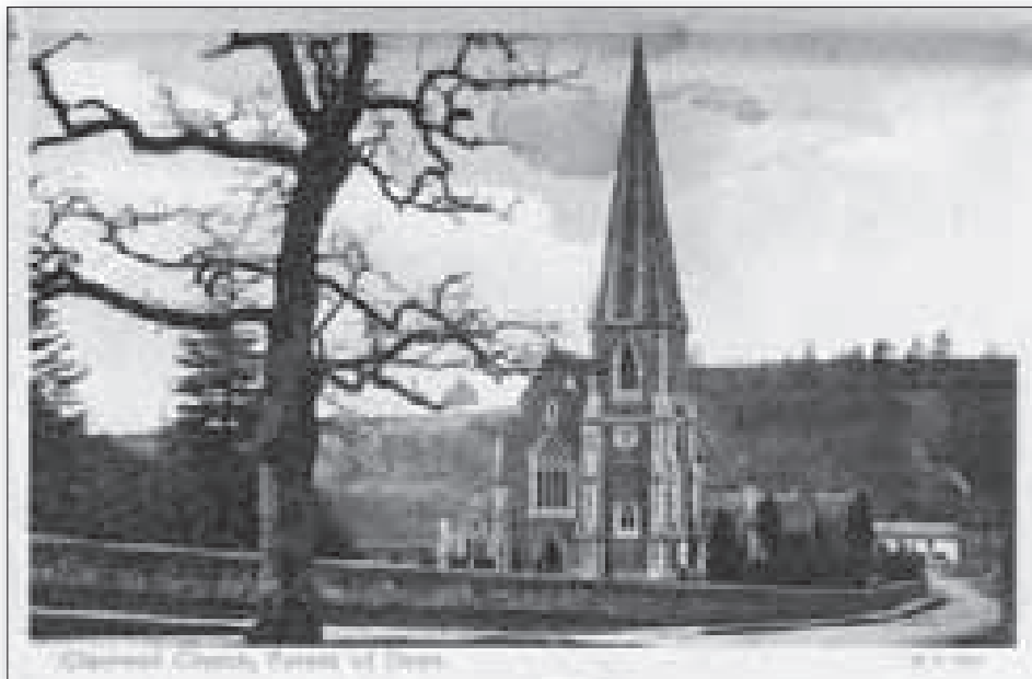
Fig. 47 Clearwell, St Peter's Church
