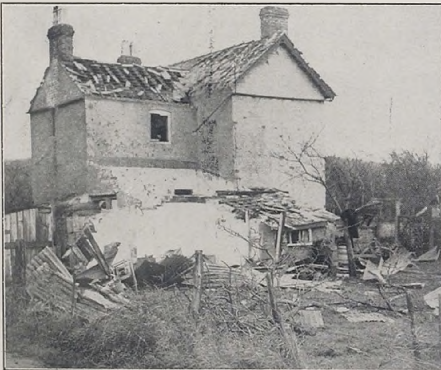
BOMB DAMAGE TO COTTAGE
