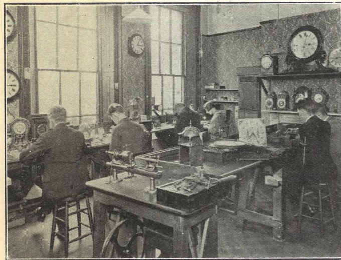
Main Workshop at 14 Clarence Street
