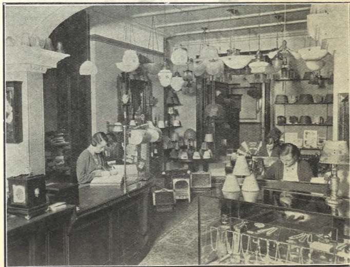
Electrical Showrooms at 14 Clarence Street
