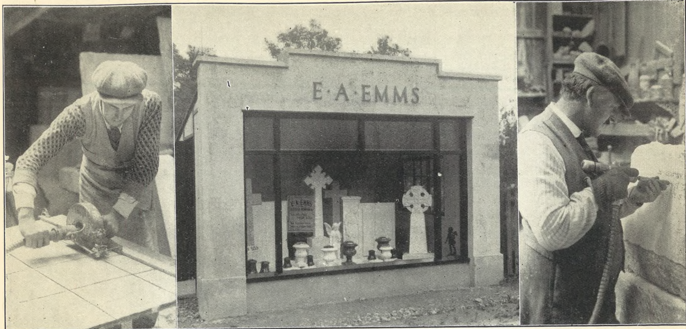
Electric Hammer drilling granite. The first process of imperishable lead lettering.
