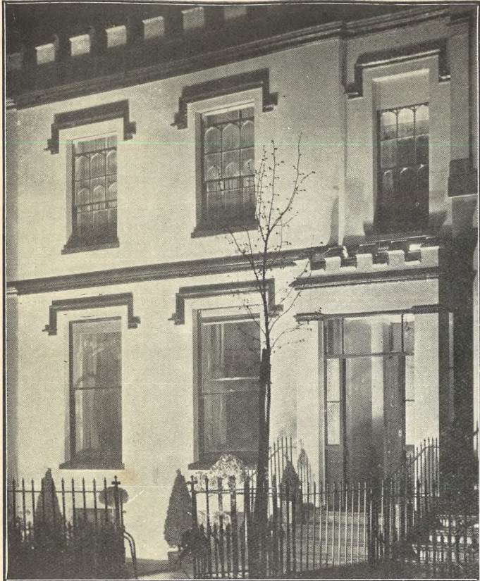
EXTERIOR FLOOD LIGHTED
