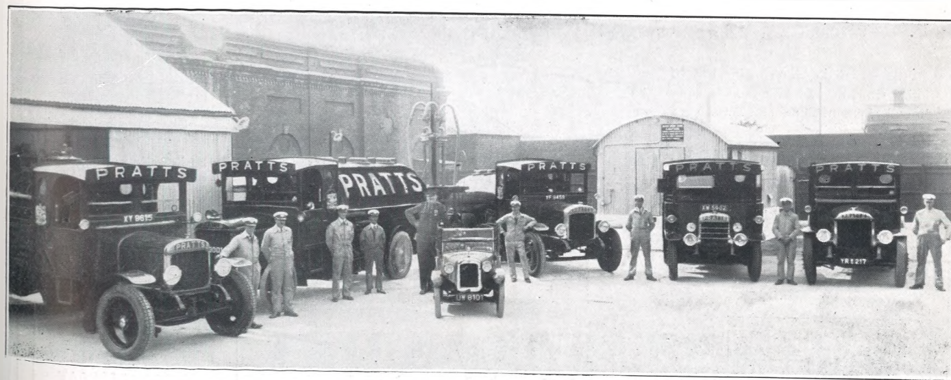
The new depot and fleet for distributing petrol and oils.
