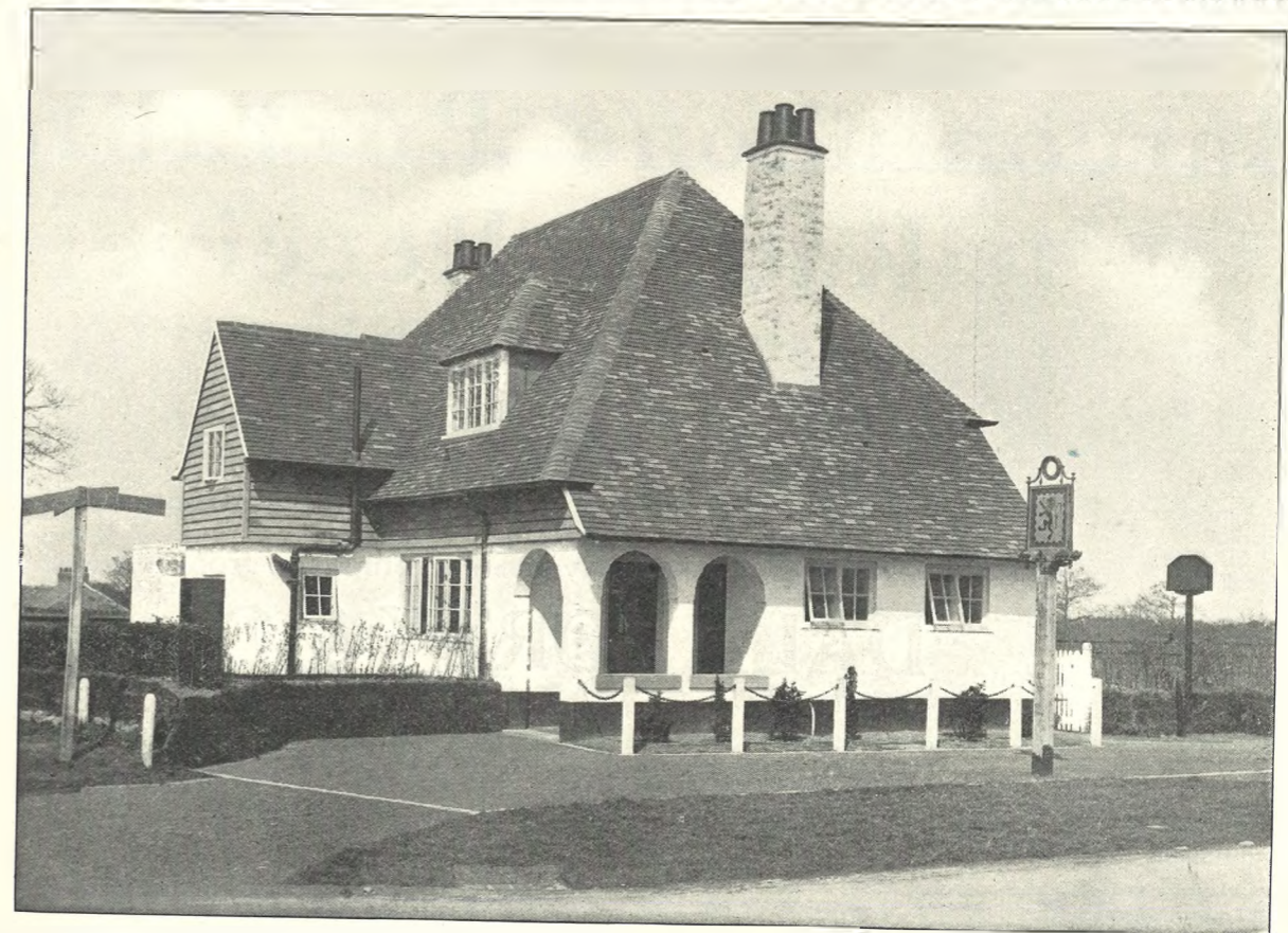
As licensed premises are reconstructed at Carlisle, Cumberland, by His Majesty's Office of Works. "Battledown" (Cheltenham), Hand-Made Roof Tiles are frequently specified. A recent instance is shown in above picture of "The Black Lion," Carlisle. The manufacturers, Messrs. Webb Bros., Ltd., are naturally proud of having His Majesty's Government as customers for many years, and also for their tiles being used for Housing at Leeds, Bournville, Welwyn, and Letchworth Garden Cities; but they are equally proud of being "received in their own country," as most of the principal new houses in Cheltenham and on the Cotswolds have been roofed by them, and they have also been adopted for Cheltenham Housing Schemes at St. Mark's and Whaddon-road.
