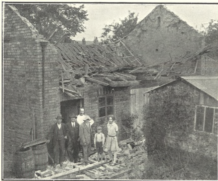
LECKHAMPTON "EARTHQUAKE." On Saturday morning, July 27, residents in Leckhampton thought an earthquake had occurred, when a large stable in the grounds of Gladstone Villa suddenly collapsed with a tremendous crash. The roof was too heavy for the weak supporting wall, which fell outwards. The house adjoins the Malvern Inn. Scene just afterwards.
