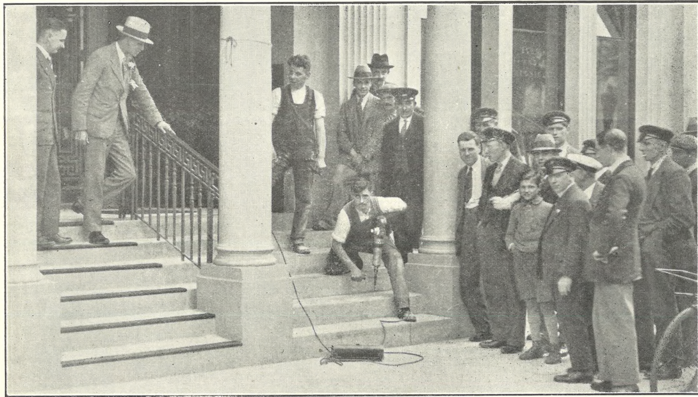
An interesting photograph of the main entrance to the "Echo" Offices showing the Ferodo Non-Slip Safety Stair Tread being fitted to the steps. On the left it will be noticed that the Stair Treads have already been fitted, while on the right the workman is drilling the necessary holes for rivetting into the stone.
