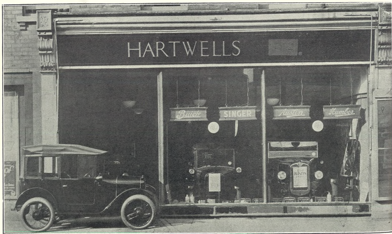
HARTWELL'S GARAGE, NORTHGATE STREET, GLOUCESTER.
