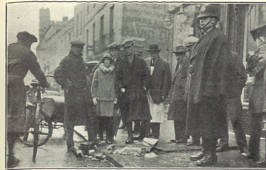
GAS EXPLOSION IN THE HIGH STREET. Shopkeepers and pedestrians in High Street, Cheltenham, had an alarming experience shortly after 10 o'clock on Saturday morning, when, owing to an accumulation of gas, the tops of two manholes were blown off, smashing the paving stones. The photo was taken 15 minutes after the explosion, showing the broken lid of the manhole opposite to Mr. Hancock's shop.
