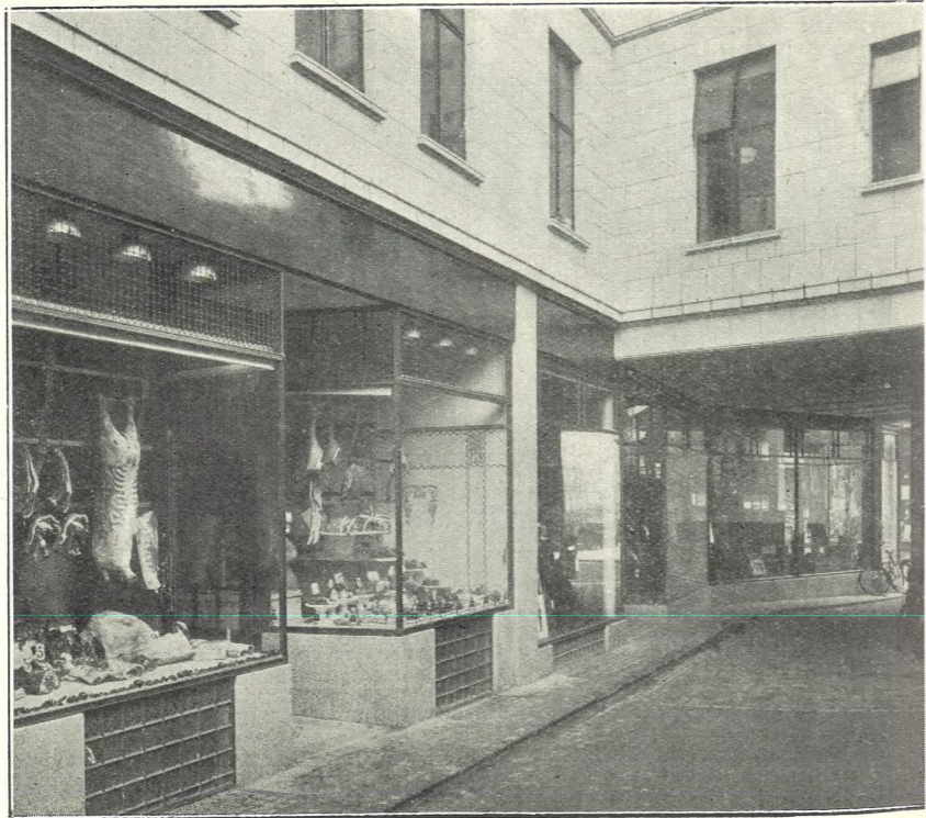
BUTCHERS' SHOP, FURNISHING AND HARDWARE DEPARTMENTS, AND ENTRANCE FROM GROSVENOR PLADE SOUTH.
