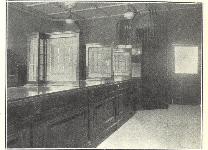
PART OF OFFICE, SHOWING CASH TUBES.
