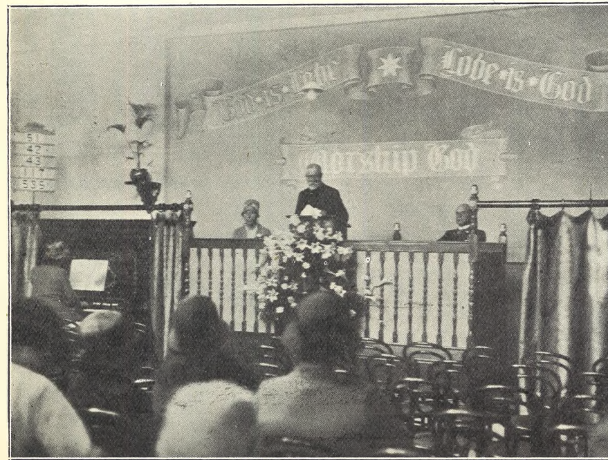
Interior of the new Spiritualist Church in Bennington-street, Cheltenham, opened a few weeks ago by Mr. H. Bubb, J.P., Ullenwood (President). It is a comfortable, well-lighted and ventilated building to hold 300 people, and contains a nice orchestral organ. Services are held at 11 and 6.30 each Sunday.
