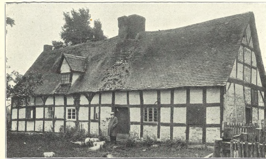
DOOMED! On Monday last the Cheltenham Town Council ordered this picturesque cottage, on the Hayden Knoll Farm estate, to be demolished. It was built in 1699. These old half-timbered cottages are one of the charms of rural England, and surely an effort should be made to save it. "Cheltenham Chronicle" Photo.
