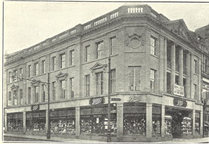
EXTERIOR OF HANDSOME NEW PREMISES.
