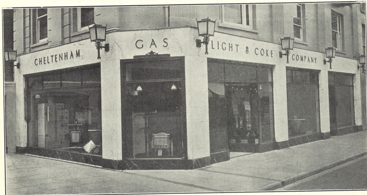
No. 40 PROMENADE (opposite the Neptune Fountain). The frontage is of Sicilian marble, relieved by black Napoleon marble. (Architects: L. W. Barnard and Partners).
