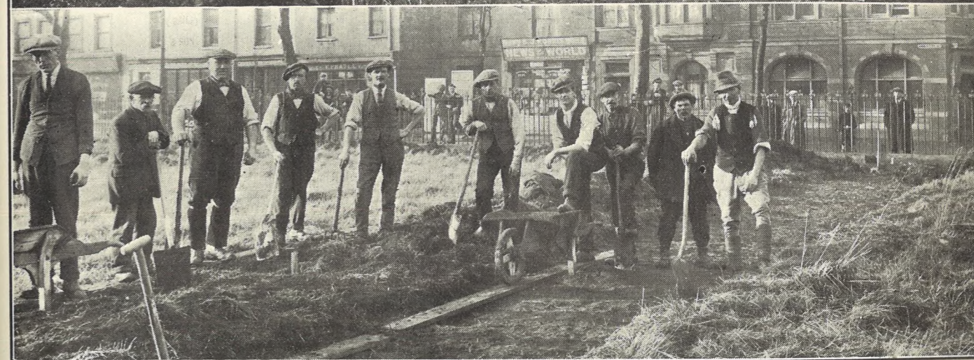
ST. GEORGE'S SQUARE IMPROVEMENT, CHELTENHAM.
