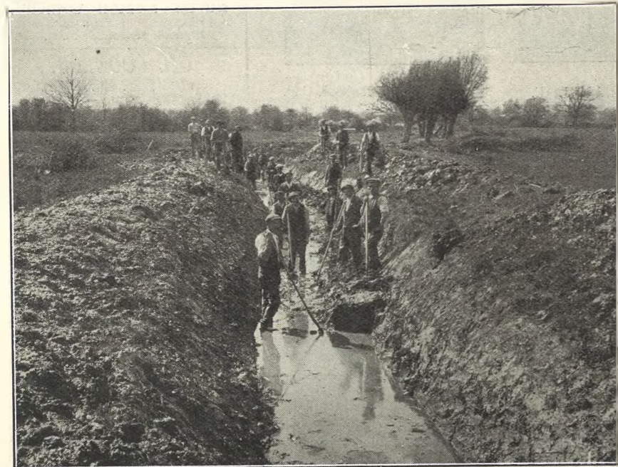
Excavating and shearing the same brook, during which many land drains are discovered and cleared after being closed up for many years.
