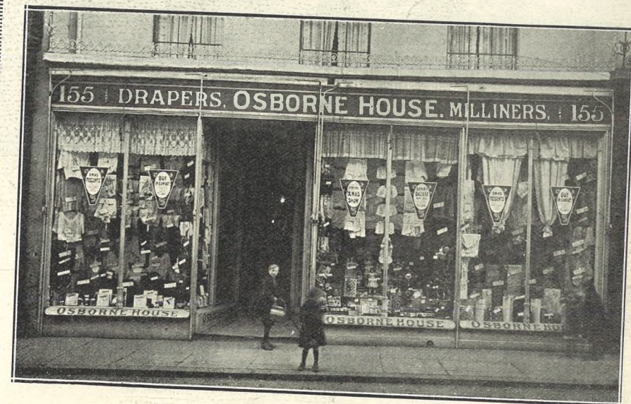
THE OLD SHOP FRONT.
