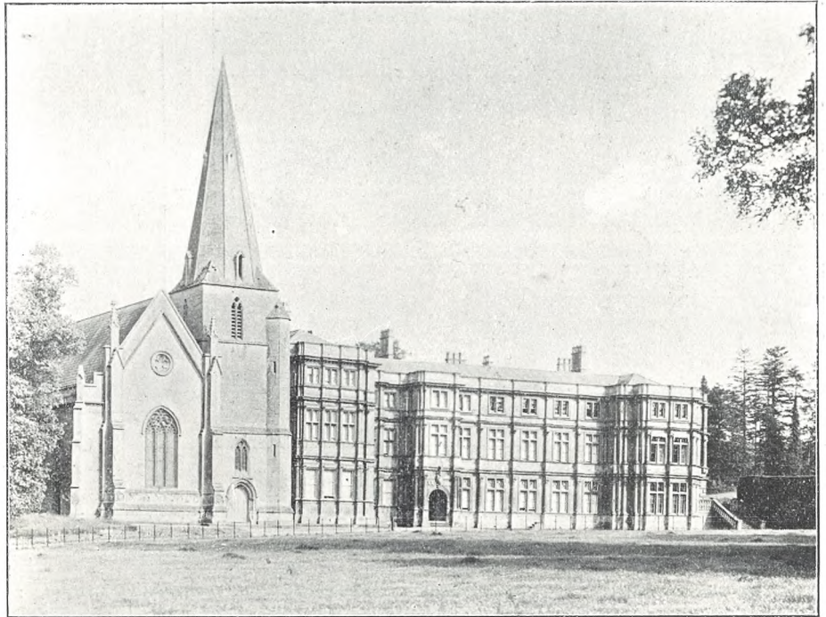
SHERBORNE HOUSE, NORTHLEACH.
