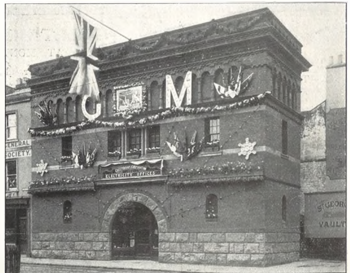
THE ELECTRIC LIGHT OFFICES, Which looked very effective when illuminated. Decorations designed by Mr. Hartnall.
