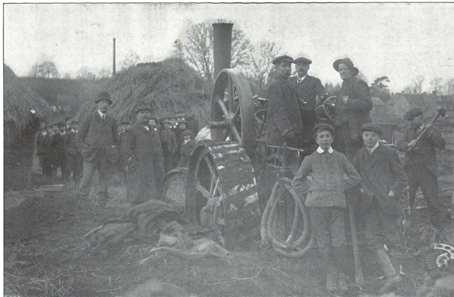
THRESHING OPERATIONS AT GREENFIELD FARM, LOWER GUITING, FEB. 10, 1910.
