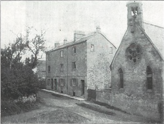
HOUSES AT BROAD CAMPDEN BUILT ON THE SITE OF HULLS'S COTTAGE BY HIS GRANDSON, RICHARD HULLS.
