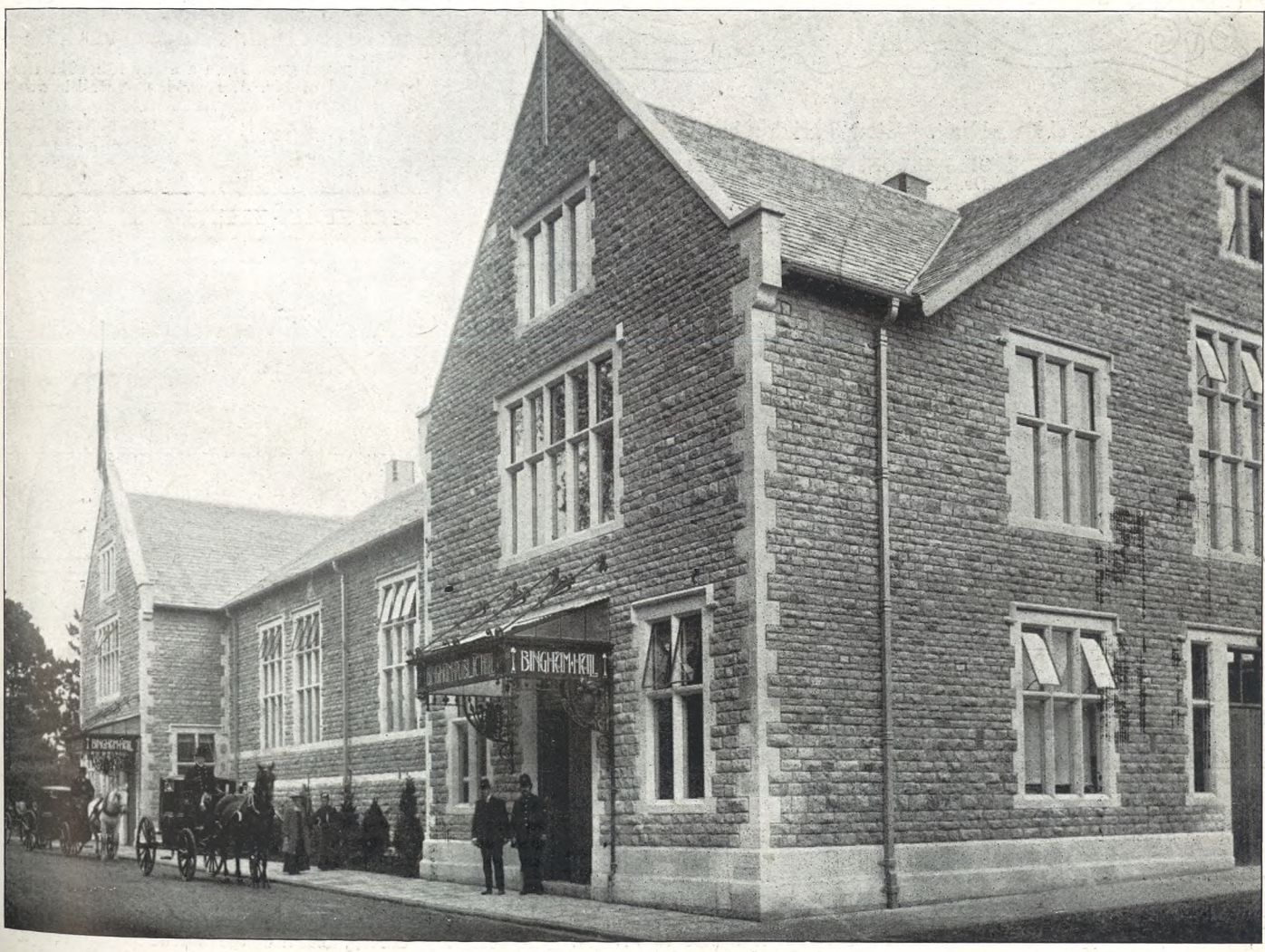
BINGHAM HALL, CIRENCESTER, OPENED OCTOBER 14, 1908. VIEW LOOKING UP KING STREET.
