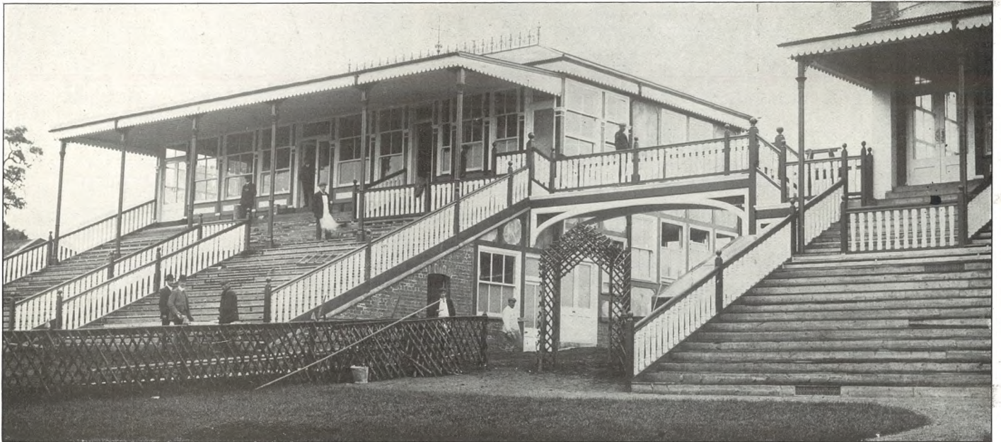
THE NEW STAND, SHOWING BRIDGE CONNECTING WITH CLUB STAND. (Designed by Messrs. Chatters and Smithson, built by Messrs. Billings and Sons, Cheltenham.)
