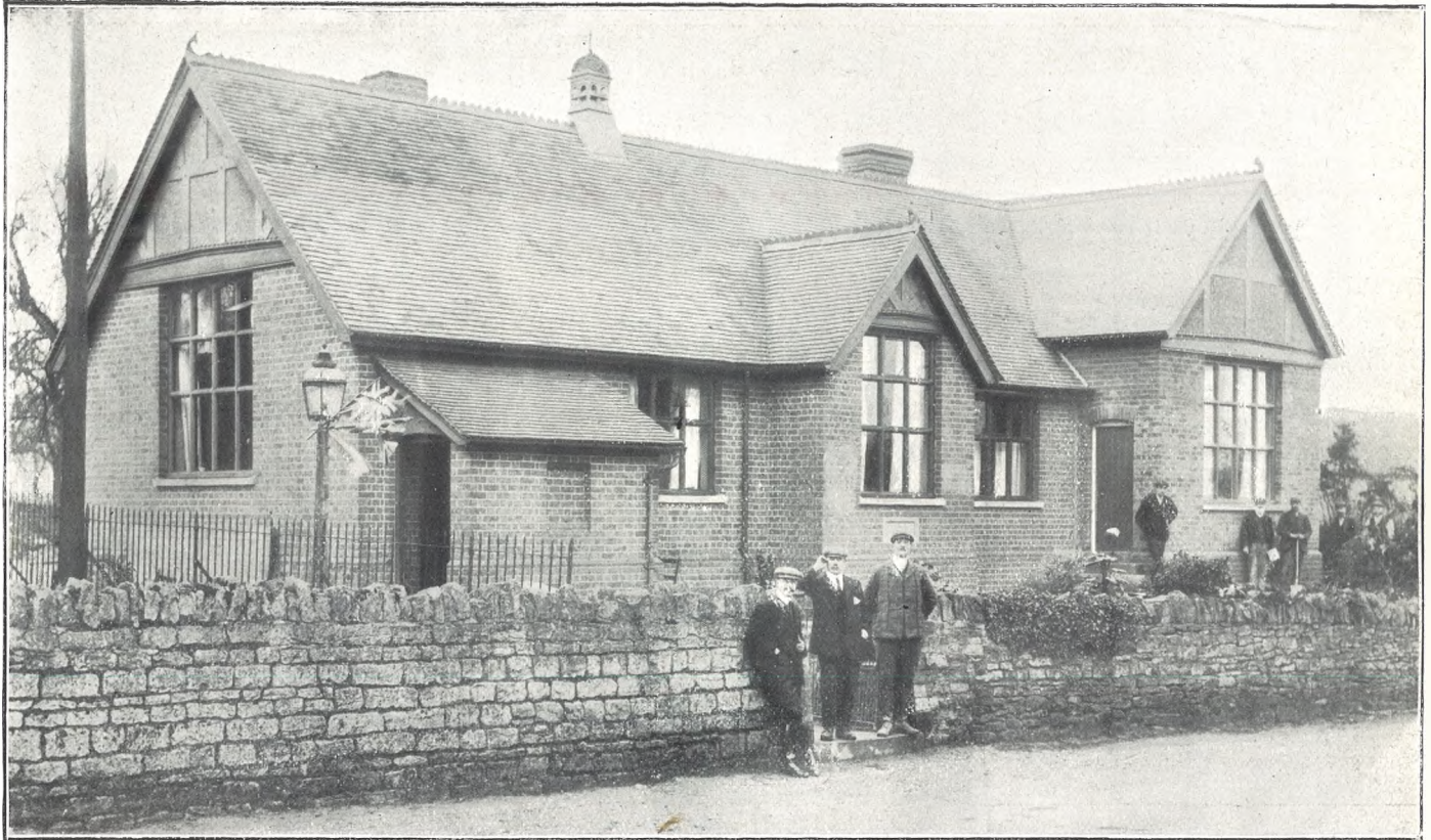
VICTORIA HALL, KEMERTON, SHOWING EXTENSION.
