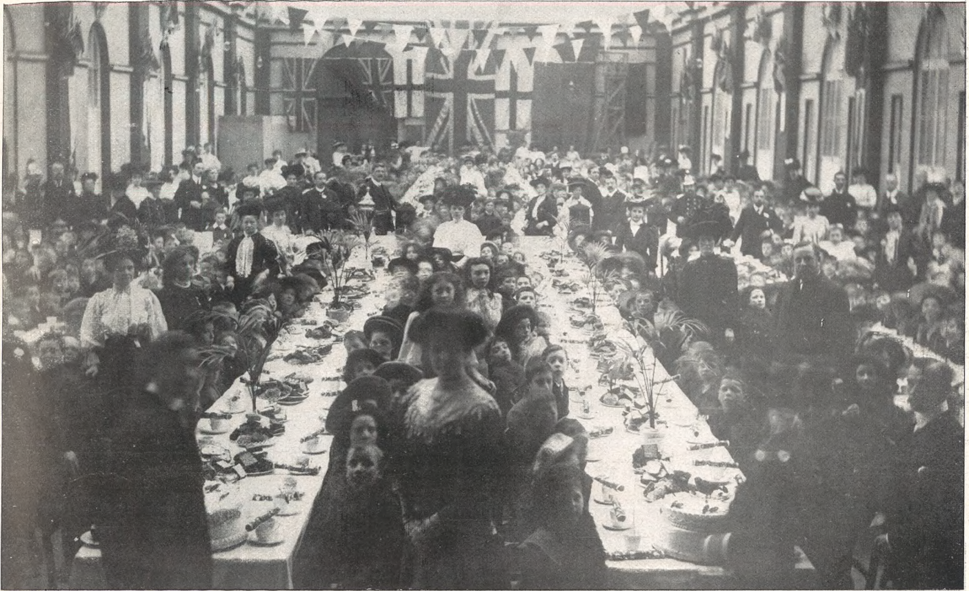
CHILDREN SEATED. GENERAL VIEW OF BUILDING.
