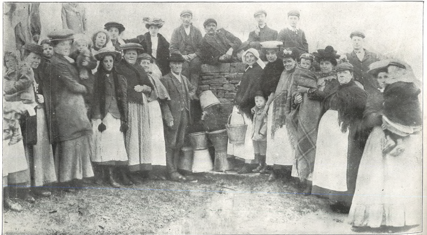
PARISH PUMP IN GRANGE HILL ROAD.
