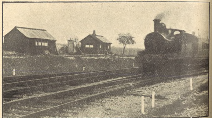
STORES AND OFFICES.—MID-DAY EXPRESS.
