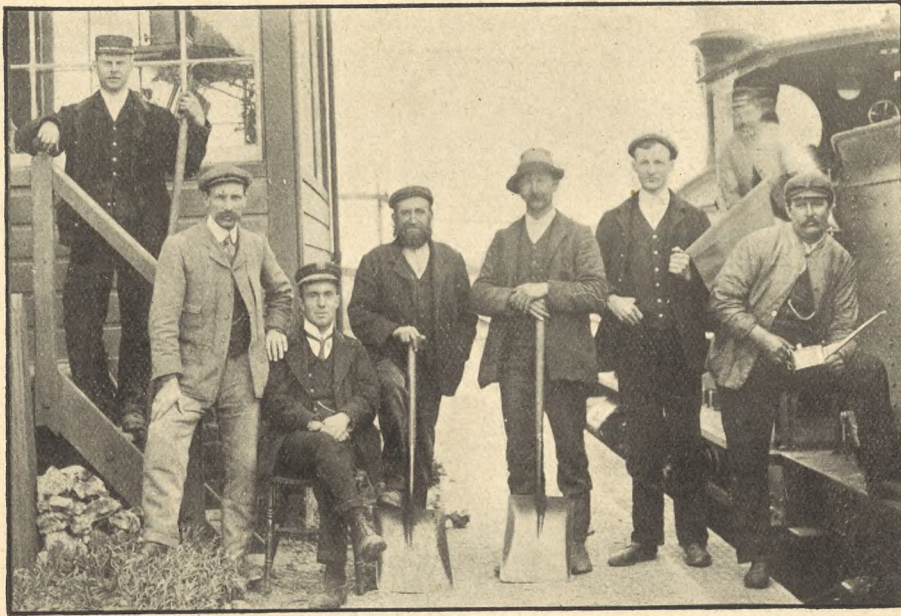
WORKERS AT FOSS CROSS STATION.
