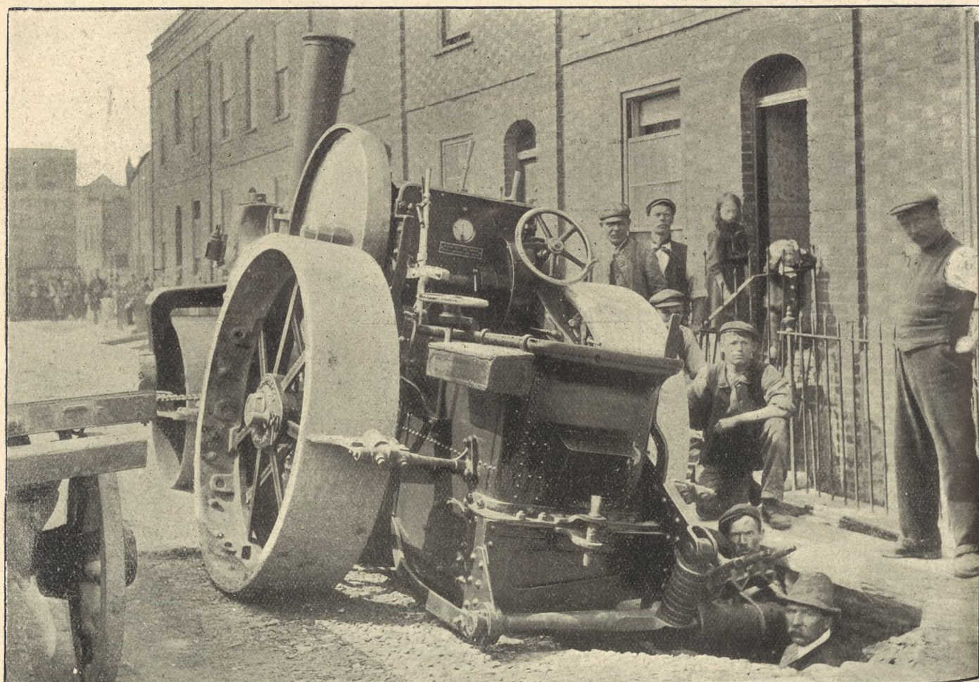
COLLAPSE OF A CELLAR IN ST. PAUL'S STREET SOUTH, CHELTENHAM, ON MAY 11, 1907, AND FALL OF A STEAM ROLLER INTO THE HOLE.
