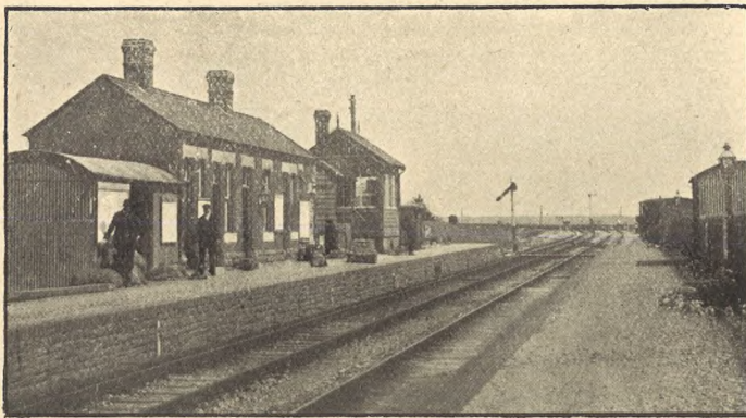
FOSS CROSS STATION, M. AND S.W.J. RAILWAY. (14 Miles from Cheltenham).
