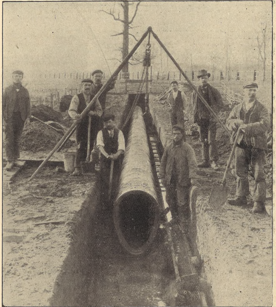
SEWERAGE WORKS AT PITTVILLE. SUBSTITUTING CONCRETE PIPE FOR BRICK SEWER.
