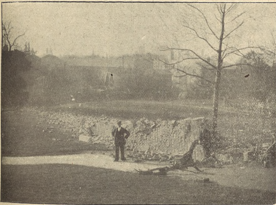
CHIMNEY AFTER FALL. Railings near tree were broken by the top stones.
