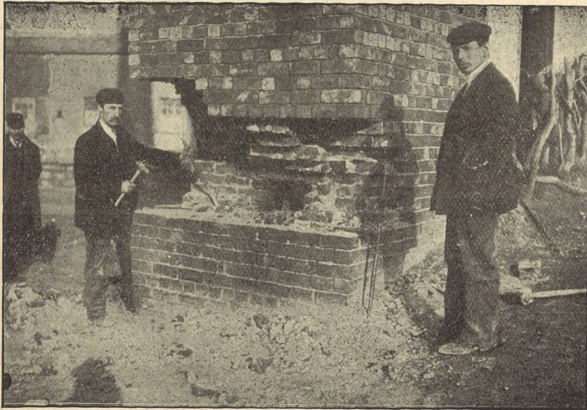
STEEPLEJACKS WORKING AT BASE. Shows how chimney was cut away.
