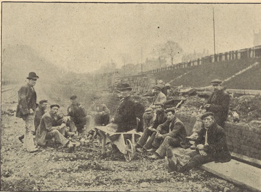
GANG OF MESSRS. SCOTT AND MIDDLETON'S MEN AT DINNER ON SITE OF NEW PLATFORM.
