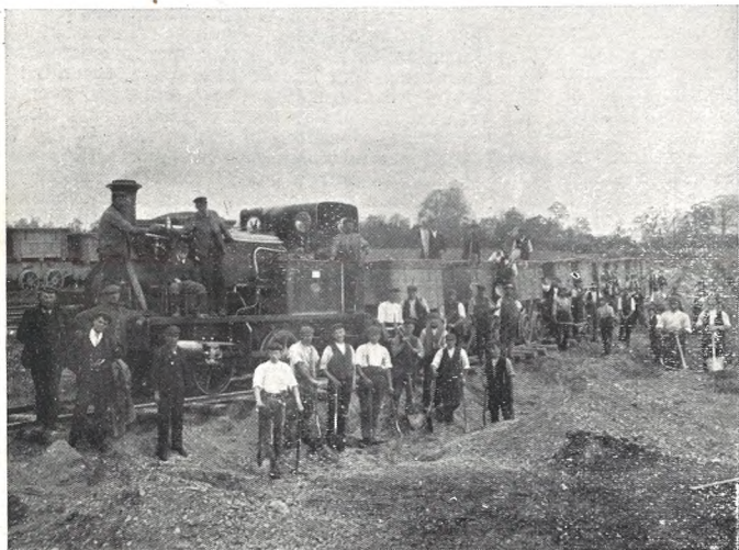
GRAVEL PITS ON THE ESTATE OF MR. E. CLIFFORD AT FRAMPTON-ON-SEVERN FROM WHICH GRAVEL IS BEING TAKEN FOR NEW DOCK AT AVONMOUTH BEING MADE BY SIR JOHN AIRD.
