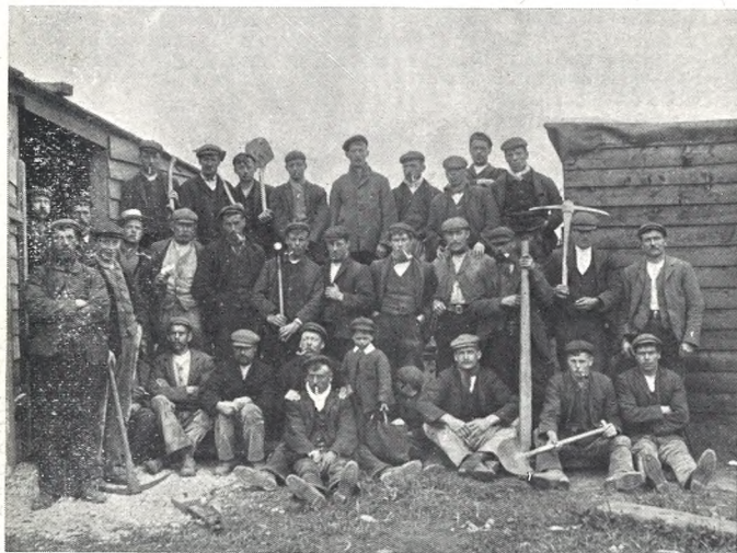
GANG OF NAVVIES EMPLOYED AT FRAMPTON.
