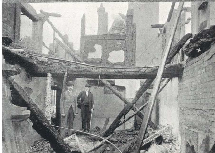
BIG FIRE AT BADGEWORTH. MAJOR SELWYN-PAYNE'S NEW RESIDENCE BURNT OUT. BEFORE AND AFTER.
