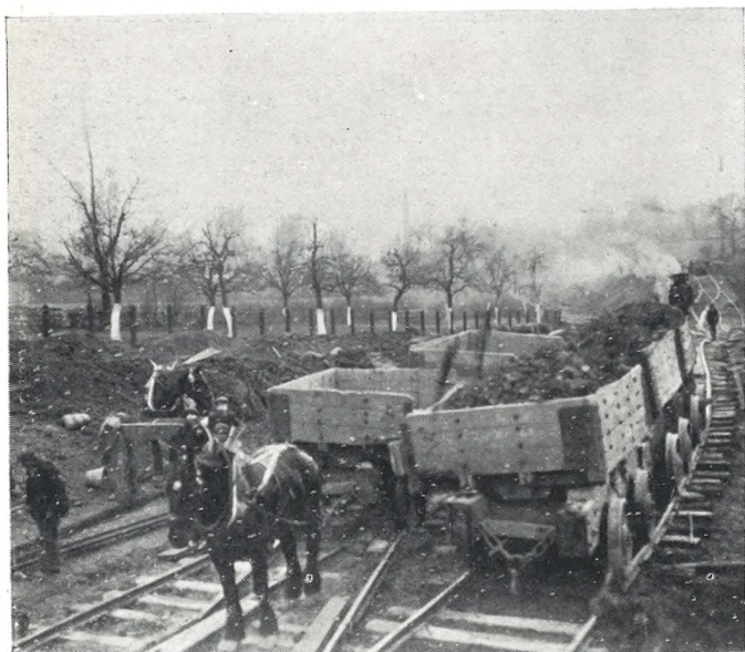
MAKING NEW RAILWAY TO HONEYBOURNE, NEAR SWINDON LANE. (Looking towards Cheltenham).
