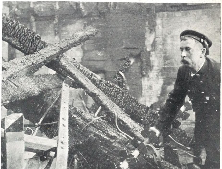
VIEW OF FIRST FLOOR WITH FALLEN BEAMS AND MACHINERY.
