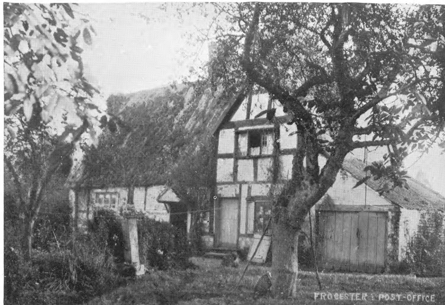
Photo by F. Restall, Stonehouse.
