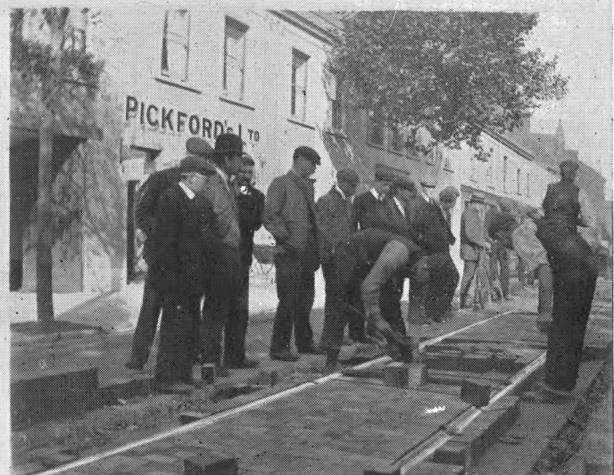
CEMENTED TRACK NEAR DICKS'S. LAYING WOOD BLOCKS IN AMBROSE-STREET.
