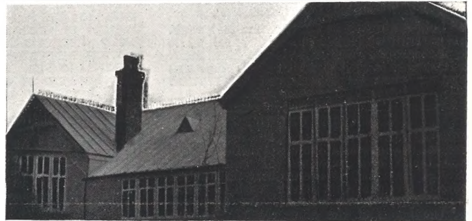
THE NEW "WINGS" AT THE BACK OF CLUB HOUSE.
