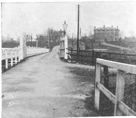
THE GATE THAT WAS BROKEN OPEN TO ENFORCE RIGHT-OF-WAY.
