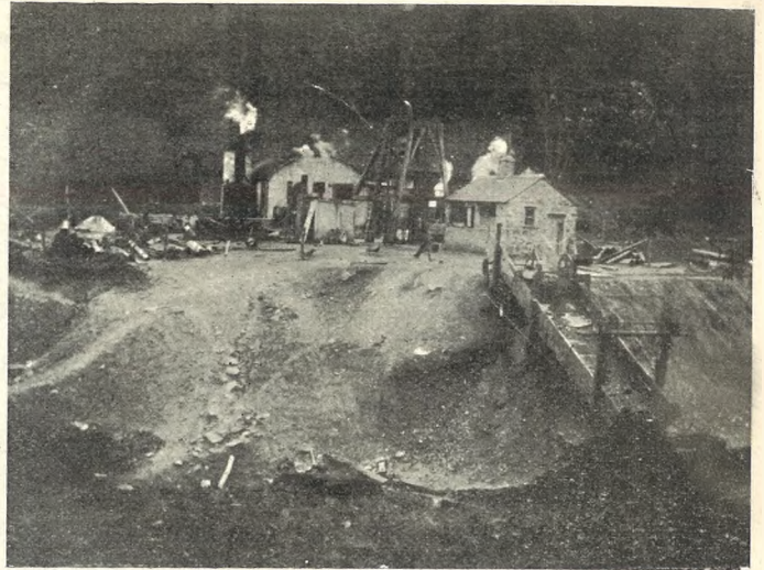
Union Pit of the Deep Navigation Coal Co Ltd., which was recently flooded and in which four miners were drowned.
