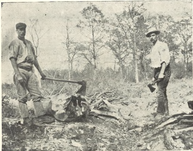
CLEARING BENHALL WOOD,
