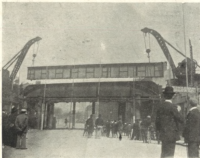
REMOVING AN OLD GIRDER.
