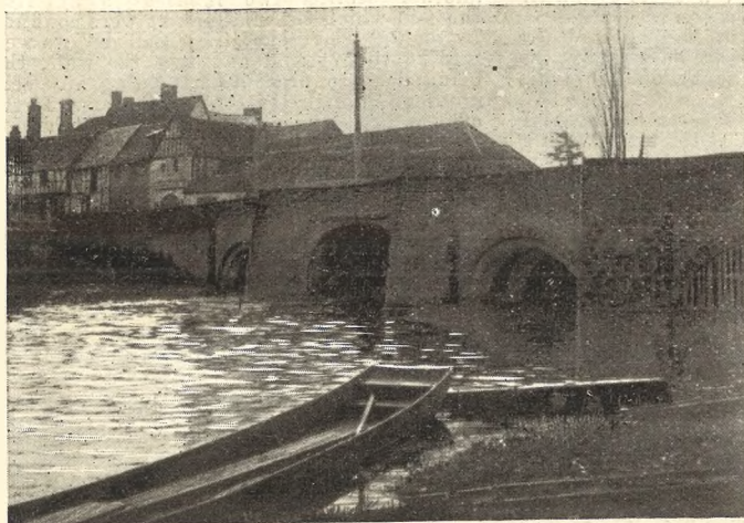
Photo by J. Willis, Prince Edward House, Tewkesbury.
