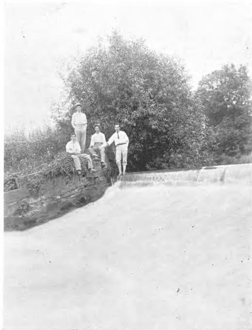
Weir Near Nafford Mill.
