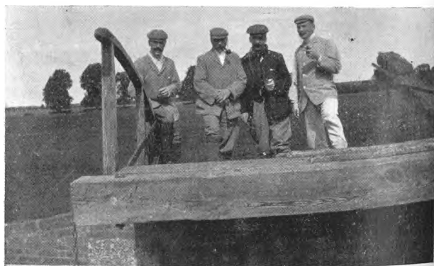
STANDING ON A BALANCED DRAWBRIDGE OVER THE OXFORD CANAL.
