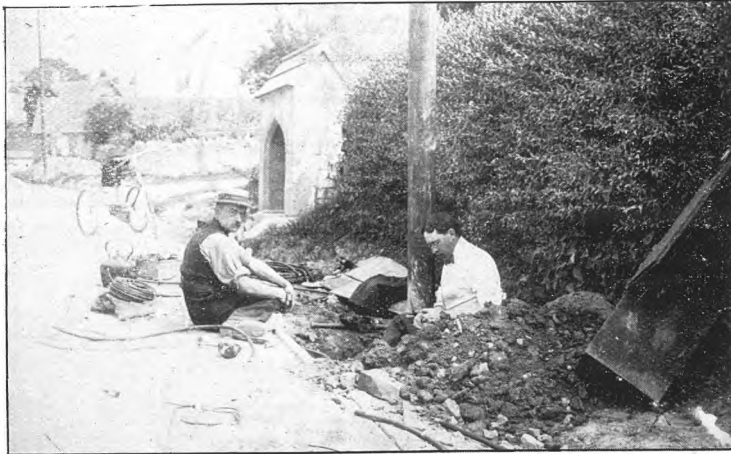
Electric Tramway—Making a Joint.
