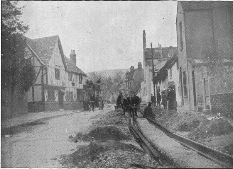
Laying the Metals at Prestbury Village.
