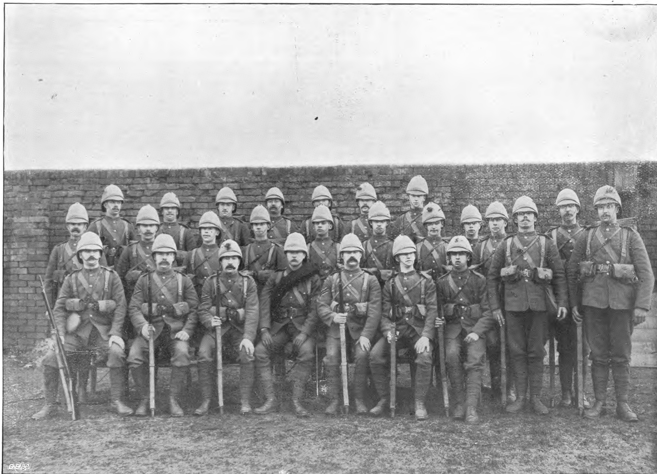
Photo by E. Debenham, Gloucester.
